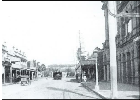
Figure 11. View south along Church Street with Post Office on right and St John's Church beyond, undated (c.1930s). 12
