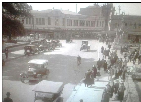
Figure 27. Northwards view along Church Street, 1938, showing Murray Brothers building at intersection. 34
