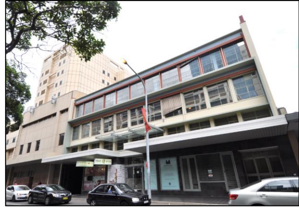
Figure 43. Marsden Street façade of addition to Murray Bros.
